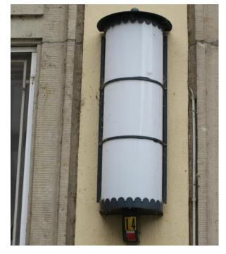
Fig. 2: This light source is part of the public street lighting network (as can be seen by the number code shown below the light). However, it does not have the classical form of a street light, and was most likely counted by the Nachtlichter participant as a "light mounted on a building".
