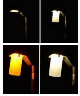
Fig. 1: Top row: Street lights without (left) and with diffusor (right). Bottom row: amber LED color temperature and neutralwhite color temperature. Photos: Martin K. Obrist, WSL
